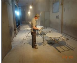
Photo of non-conformity NC 7.6 one painting worker not wear the provided gas mask and safety clothes.JPG
