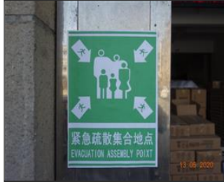
Photo of fire safety equipment Assembly point.JPG
